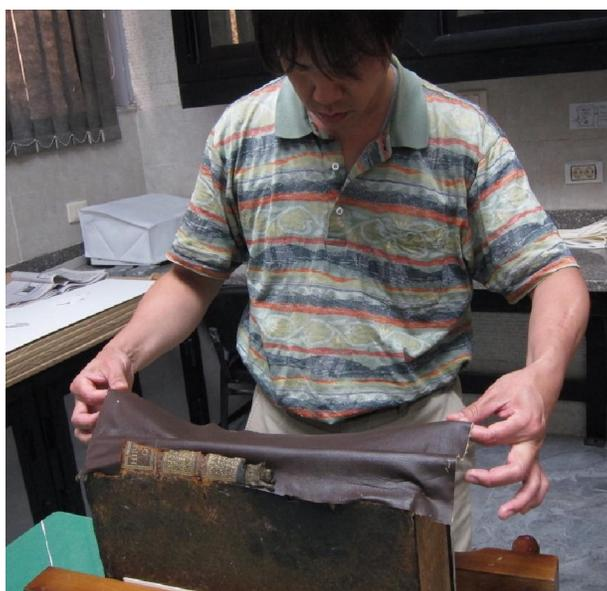
Fig. 23. Inserting the periphery of the new leather beneath the original leather.
