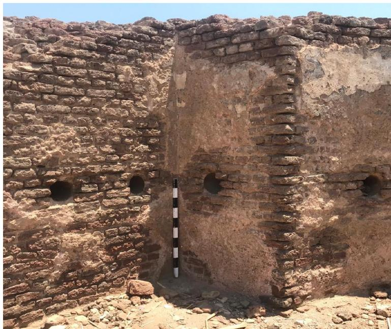
(Fig.5): A picture showing the internal cavities of the northern wall, as well as the architectural cracks in the building from the site.
